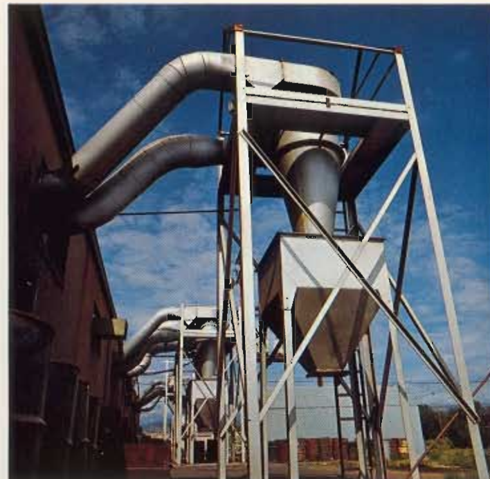
Cyclone air cleaners power dust collection system.
